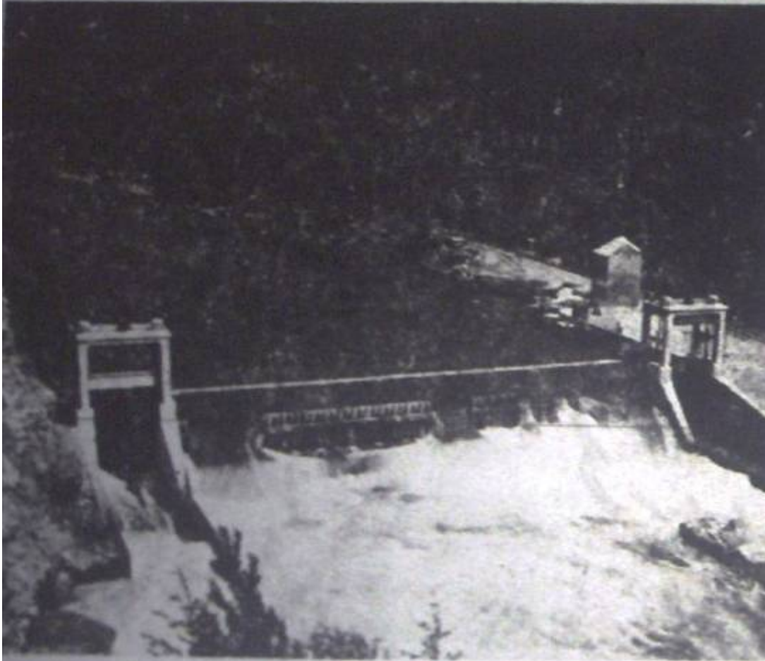
Seattle City Ligh's Gerge Diversion Dam, furthest downstream of the three, as it appeared at the start of construction on new dam.
